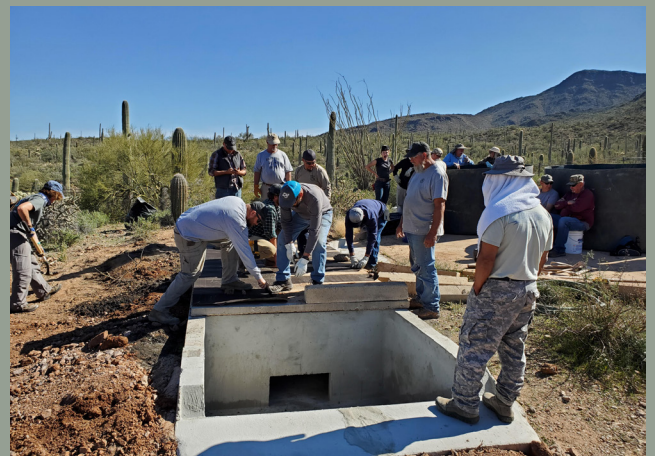
Volunteers with ADBSS install a wildlife water catchment and storage system to benefit bighorn sheep and other wildlife at Woodin Ranch.
