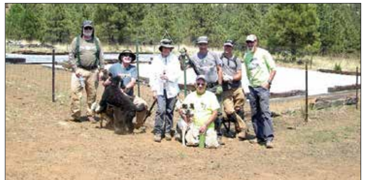
Members of the Friends of Northern Arizona Forests gather for a well-deserved photo op after completing their latest project, rebuilding a wildlife water catchment apron north of Flagstaff at Saddle Mountain.
