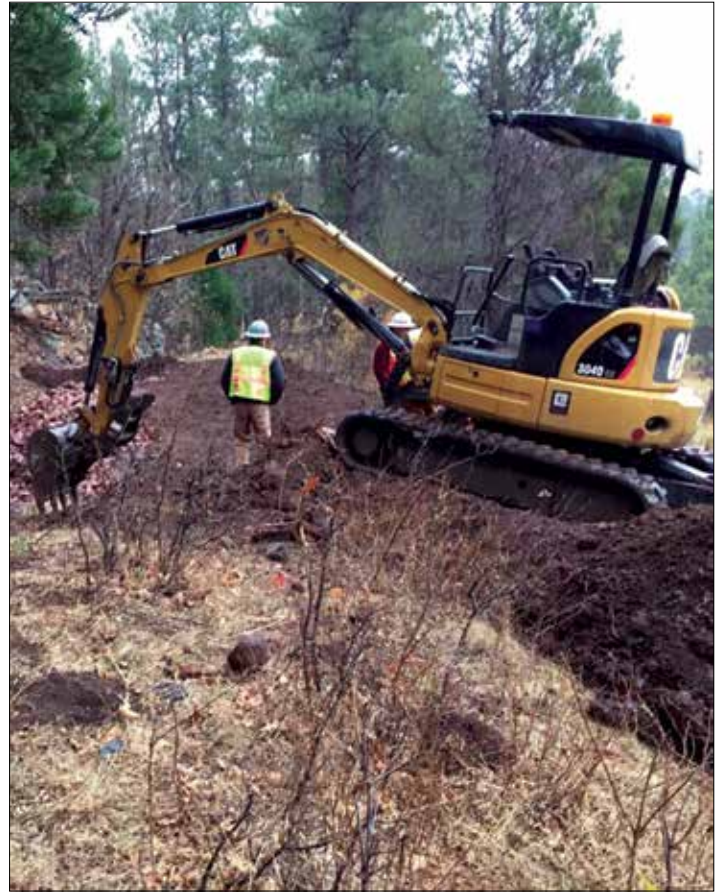
Heavy equipment working at T-Six Spring to fill in an old diversion ditch so spring flows return to their natural channel.
