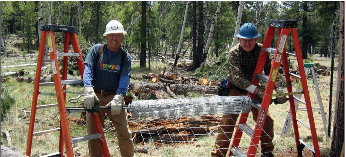
Unspooling woven wire for new fence
