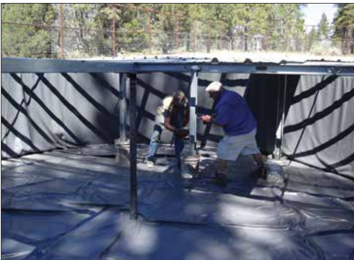
AES volunteers repair a trick tank in Unit 9
