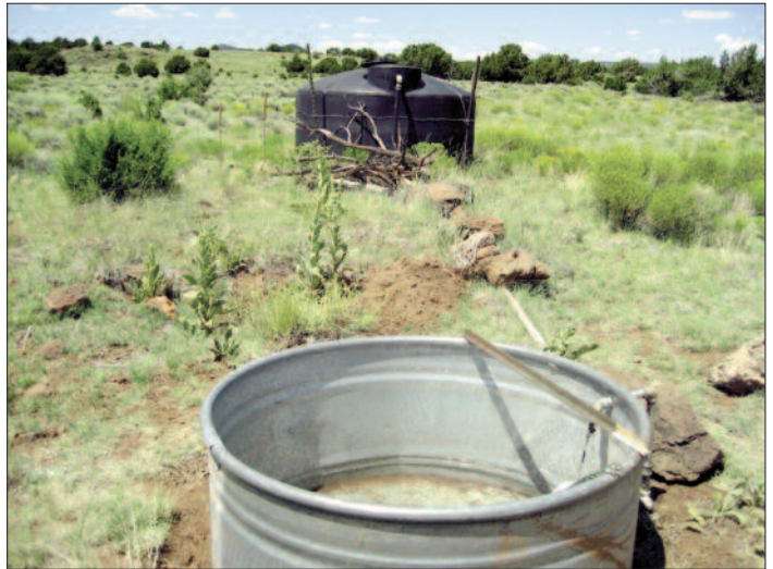
Drinker #3B on the Pat Springs Pipeline
