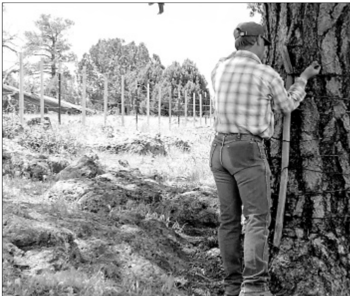
Travis Removes Old Wire
